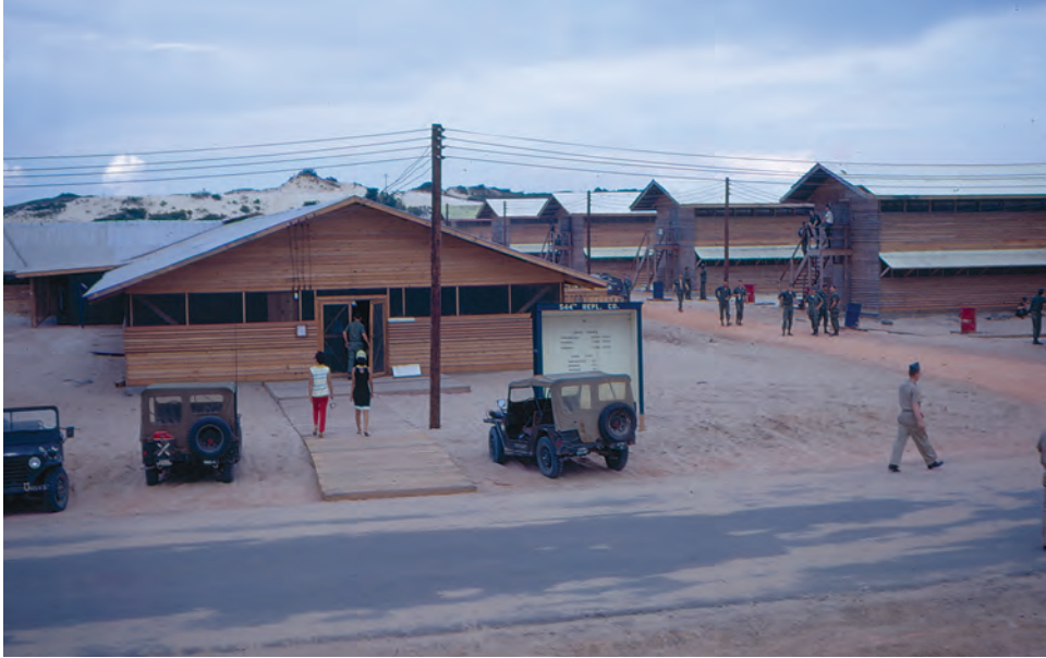
During 1968, wooden tropical barracks and administrative buildings, designed and built by the 35th Engineer Group such as these buildings in the replacement center, had replaced tents at Cam Ranh Bay.
